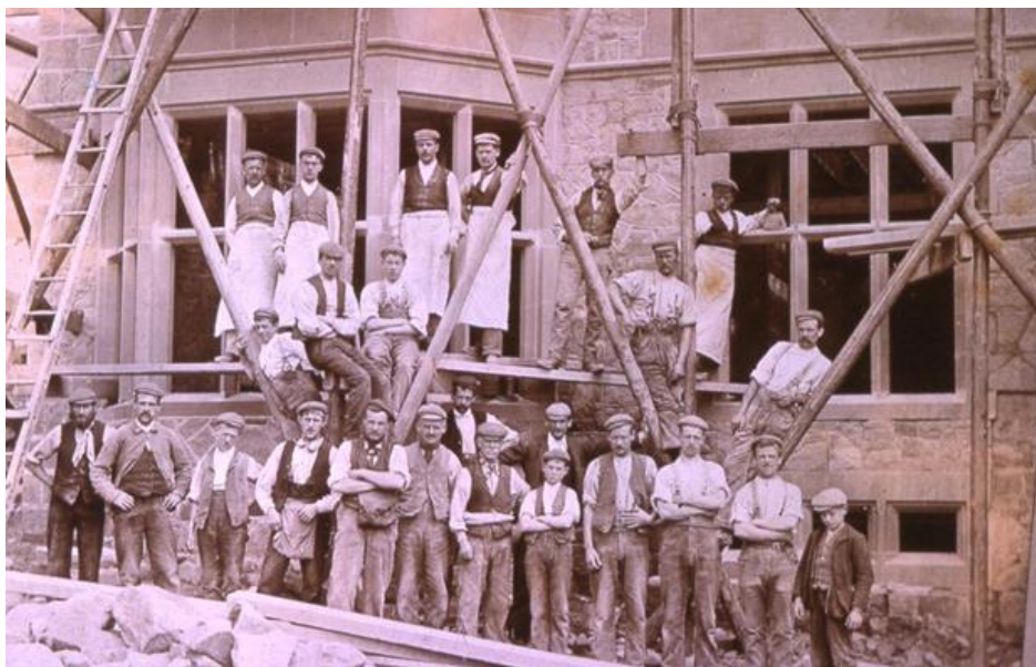
Building work at The Maynard
